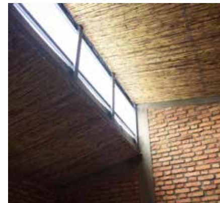
Reed Ceiling Detail |
